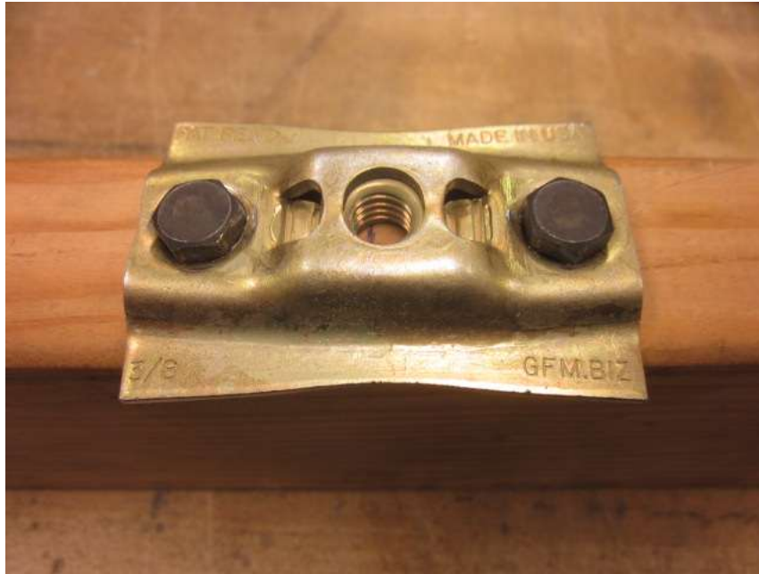
Photo No. 1 Typical Flange Plate Detail
